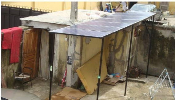
Solar Panels installation
